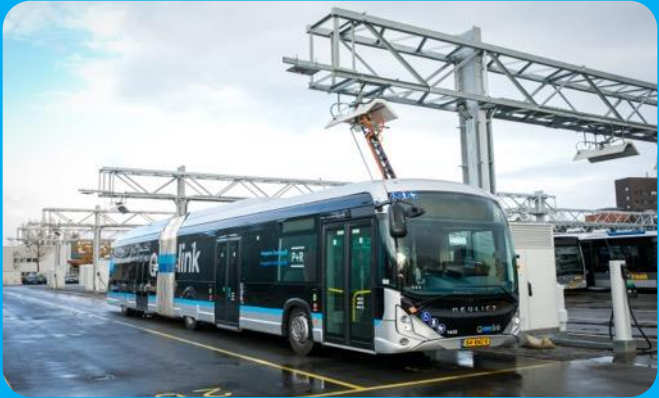
100 depot overhead chargers (50-150kW)
