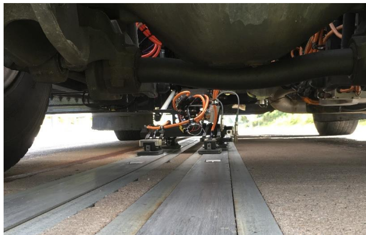
Figure 8. Dynamic charging from the ground (Alstom APS solution for ERS)
